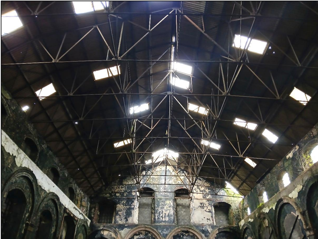
Plate 16. Steel trusses holding up the roof, showing occasional skylights and missing roof panels, looking west.
