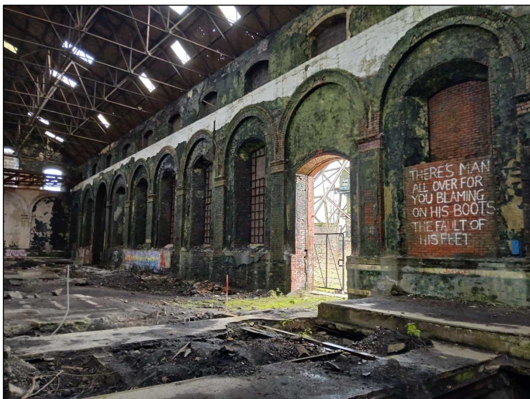
Plate 15. Example of continuous arcading along the southern side of the interior of the Engine Hall, looking southeast.
