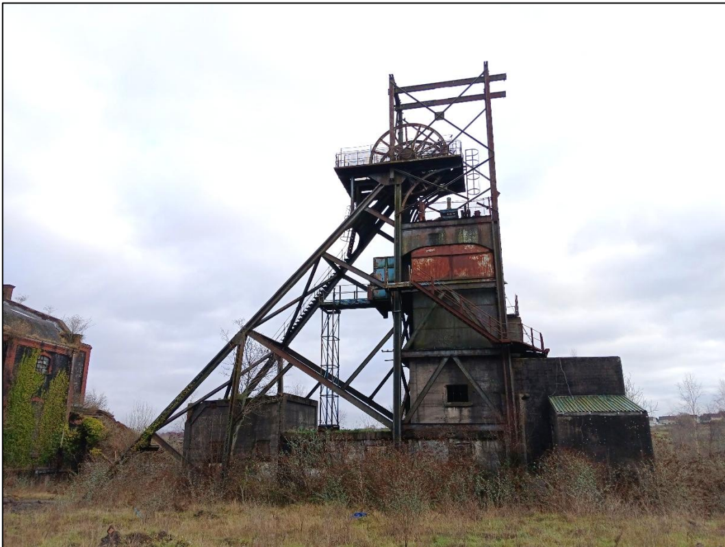
Plate 29. No. 2 Headframe of Penallta Colliery, showing concrete structures around its base, looking east.
