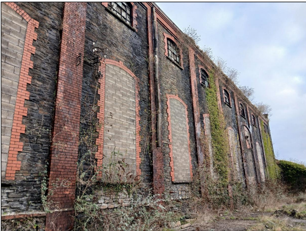
Plate 7. Examples of infilled window openings on the southern aspect of the Engine Hall, looking northeast.
