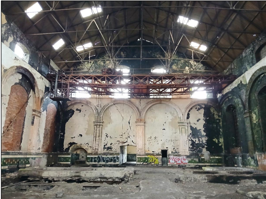
Plate 18. Eastern end of the interior of the Engine Hall, showing the lattice girder crane, looking east.
