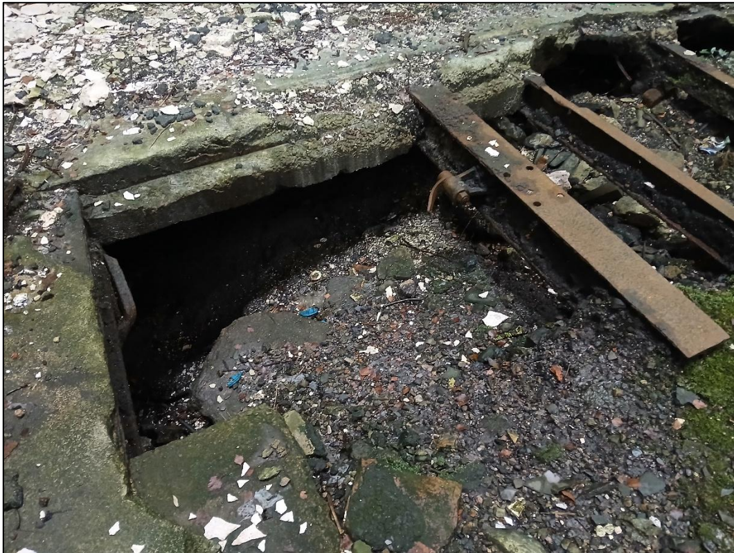
Plate 19. Example of loose material used to infill the basement of the Engine Hall, looking northwest.
